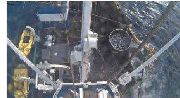
UNLOADING BRAIL WITHOUT HOPPER
